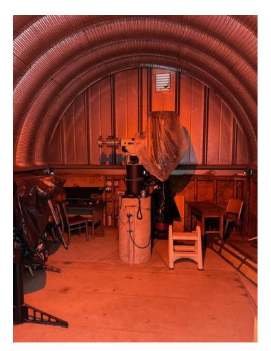
inside this peculiar-looking building. The entire roof rolls off the structure and onto the rails behind it.
