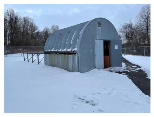
The advantage of this system is that once the roof has been moved out of the way, telescopes inside the building can now point in all directions freely; there's no need to make adjustments throughout the night as the telescope moves.
