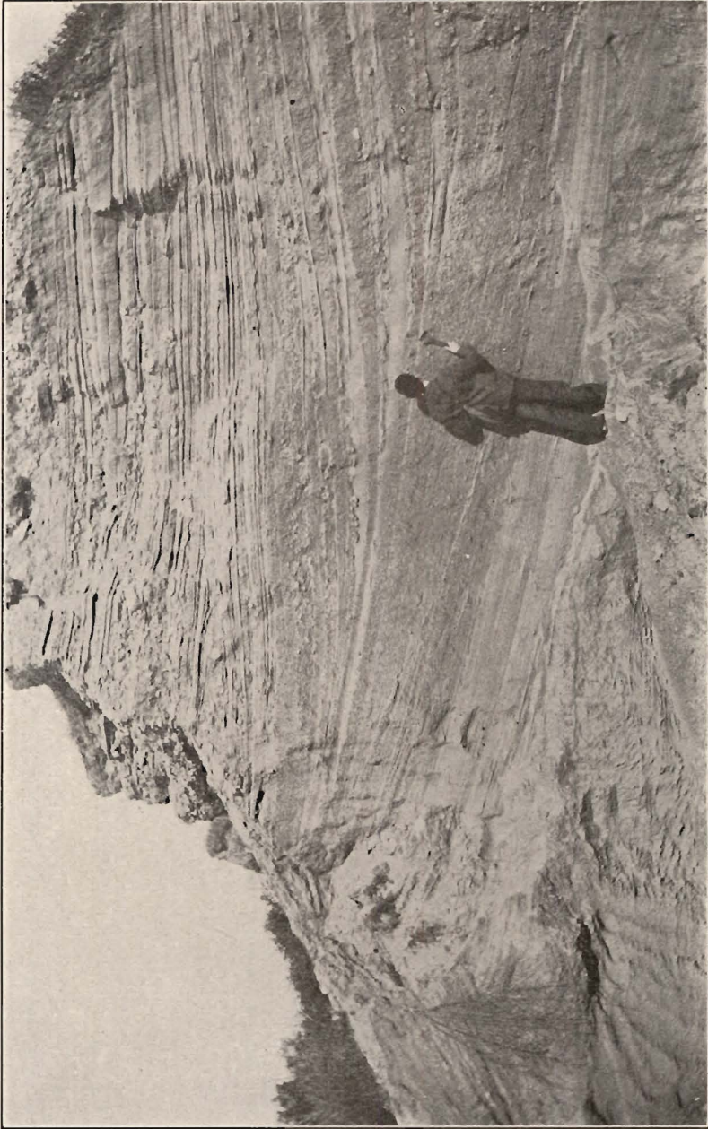
BRIGHTON EXCAVATION Sheehan pit. Alternation of fine and coarse layers
