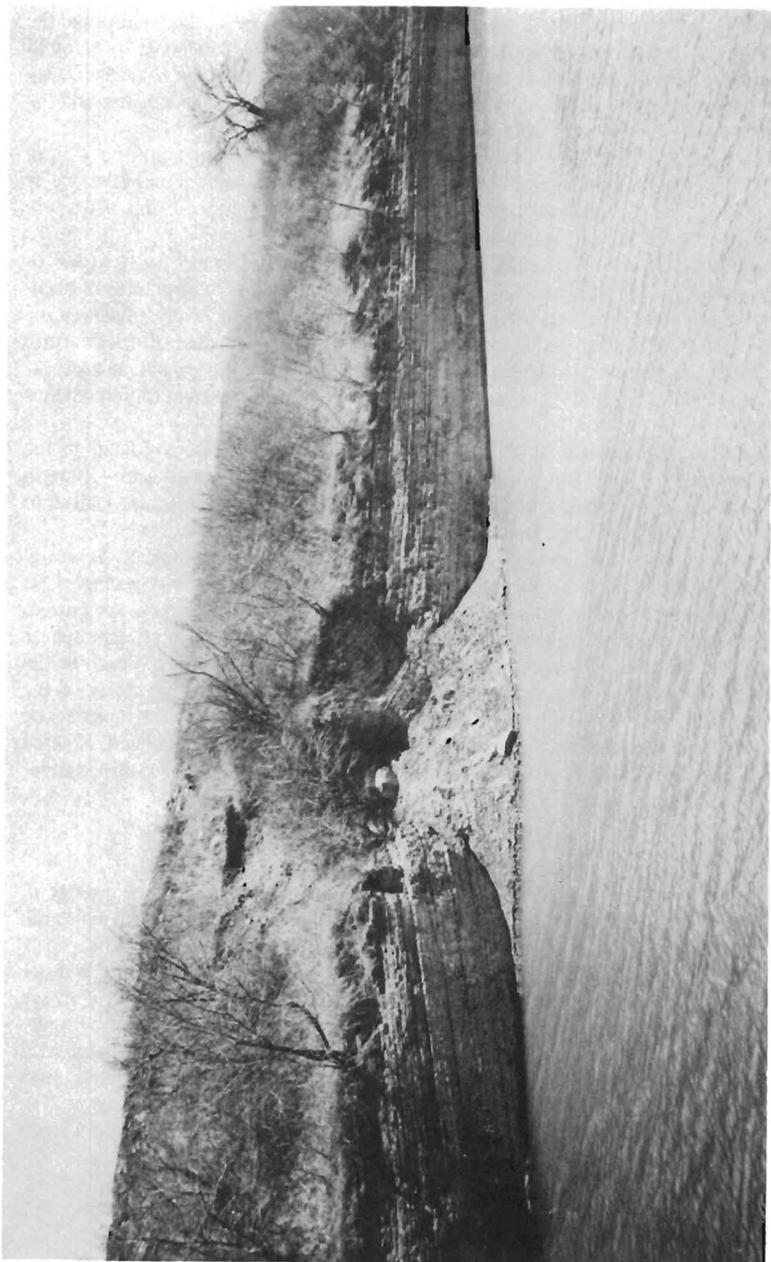
*FIGURE 7: Central portion of broad fold-fault structure visible in N. Y. State Barge Canal (structure zone A, Figure 2). View to southeast. Zone A and B are inferred to consist of numerous subparallel offsets or flexures with a maximum measured displacement of 18 feet on one fault penetrated by a boring (H & A of New York, 1981).*
